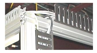
Figure 59: Wiring Channels
